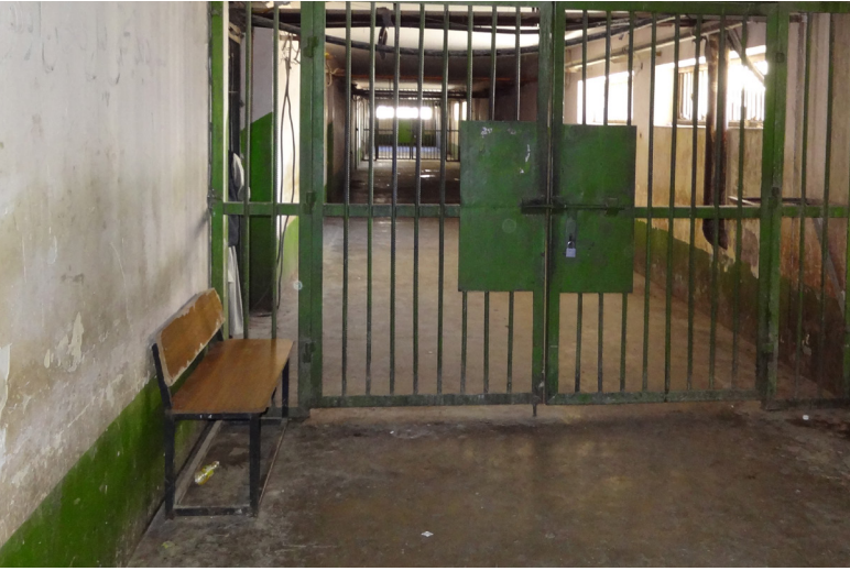
Hallway at Pol-i-Charkhi Prison. Photo: Special IG for Afghanistan Reconstruction on Flickr (CC BY 2.0)
